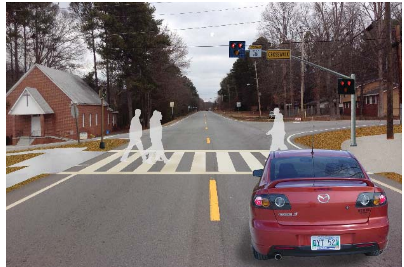
Proposed Intersection of Emory Street and Richardson Street with the Installation of HAWK beacon
